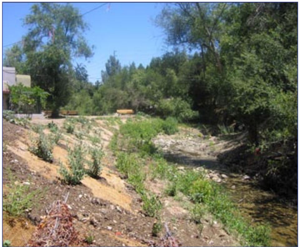
After Restoration: Gently sloping bank with riparian and wetland plants.
